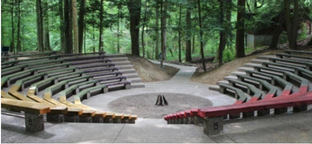
Council Circle renovations nearing completion. ▲
